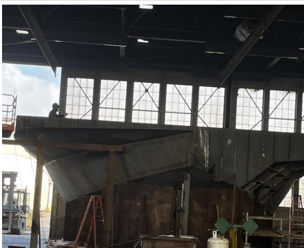
2986 – Module 1 with Bulkheads being fitted
