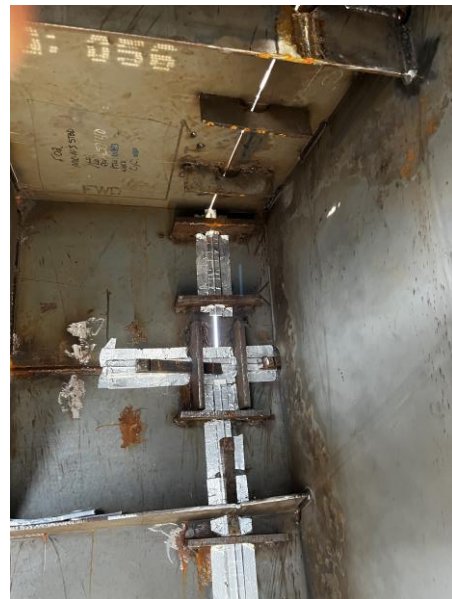
3227 – Preparation of Master Butt Joint so can weld from outside. Ceramic tape is used to help properly contain weld.
