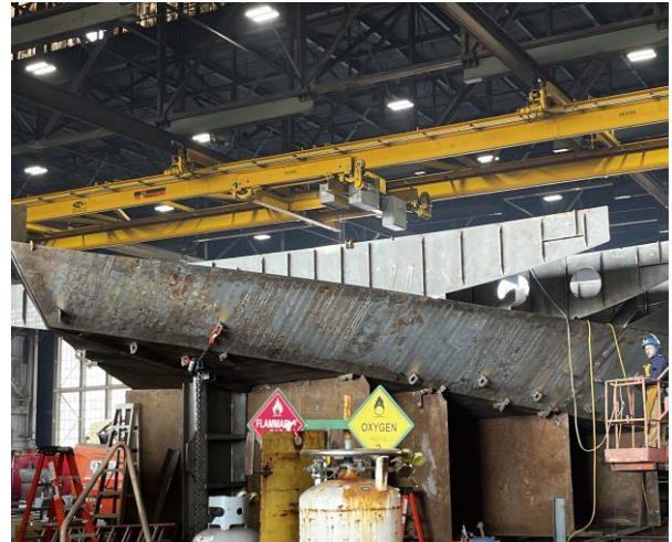
3152 - Module 5 having side shell hull plating installed
