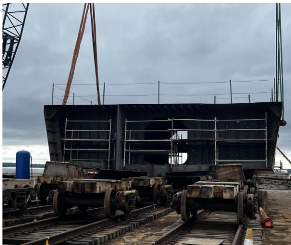
3032 – Module 3 being lifted onto the Erection Runway
