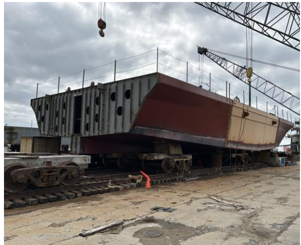
2371 – Modules 2, 3 & 4 aligned on Erection Runway
