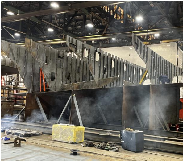
3120 – Module 5 Transverse Bulkheads in-place
