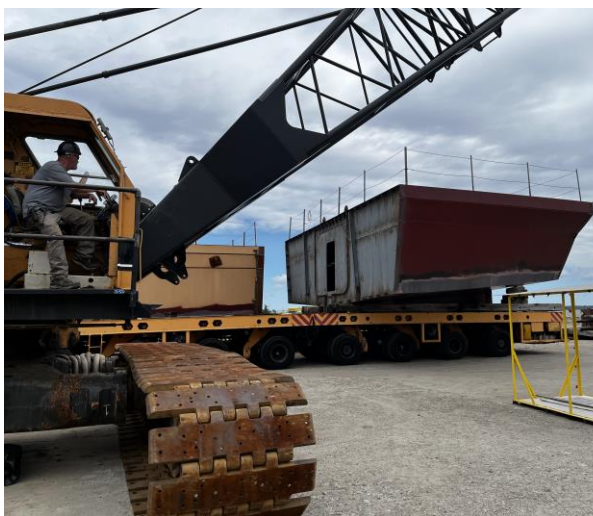
3099 – Module 2 heading for the Erection Runway
