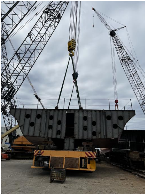
3102 – Lifting Module 2 into place on the Runway
