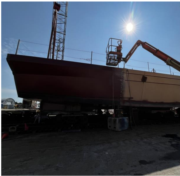
3078 – Preparing the Master Butt (seam) between modules 3 & 4
