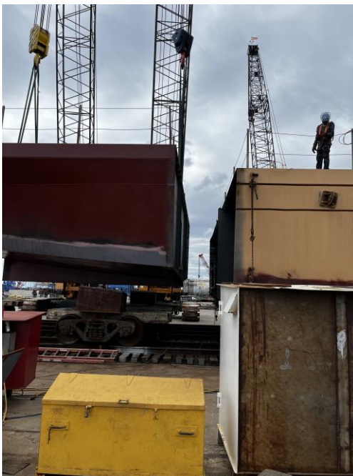
3105 - Lifting Module 2 into place on the Runway
