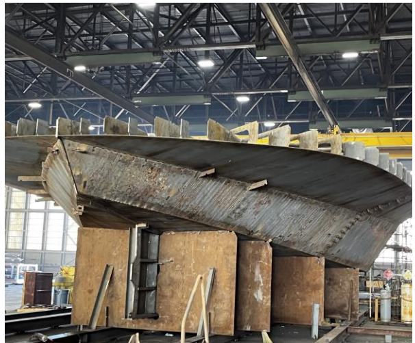
3232 - Module 5 with Guard framing in place
