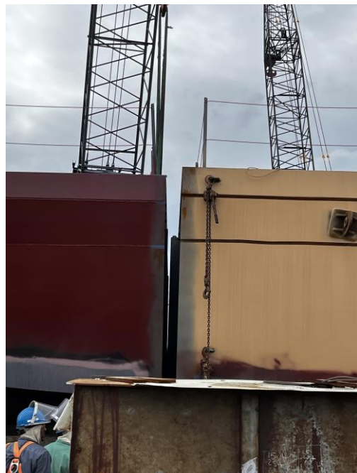
3106 - Lifting Module 2 into place on the Runway
