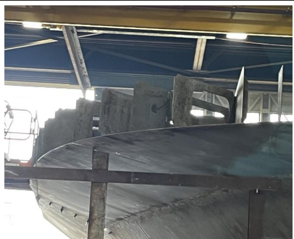
3005 – Module 1 Guard framing being installed
