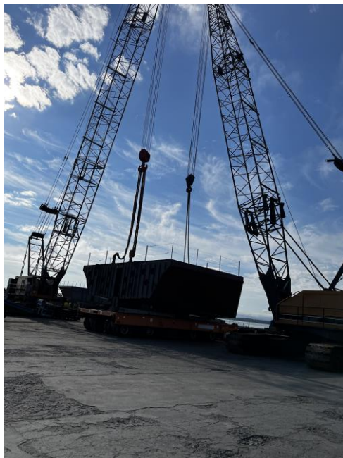
3040 - Module 3 being lifted onto the Erection Runway
