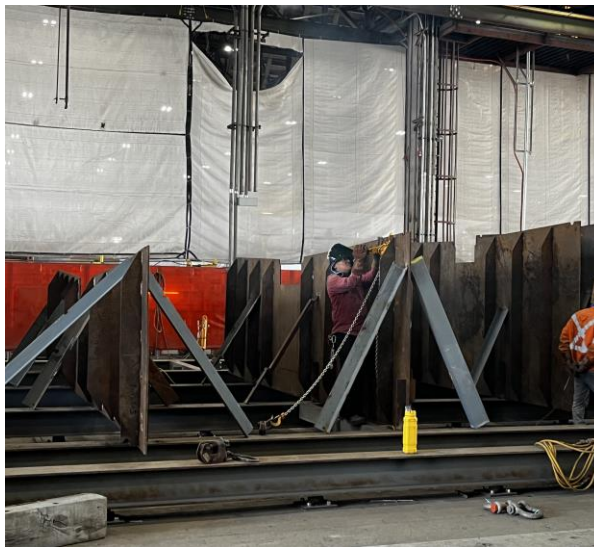
3039 – The Falsework Gig for Module 5
