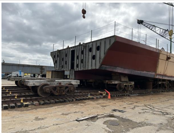
2372 - Modules 2, 3 & 4 aligned on Erection Runway
