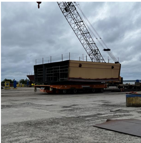
3027 – Module 3 after painting, being moved to the Erection Runway area for assembly with other modules
