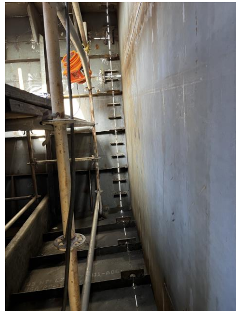
3087 – Strong Backs on the Master Butt between 3 & 4. These help hold the seam at the proper alignment
