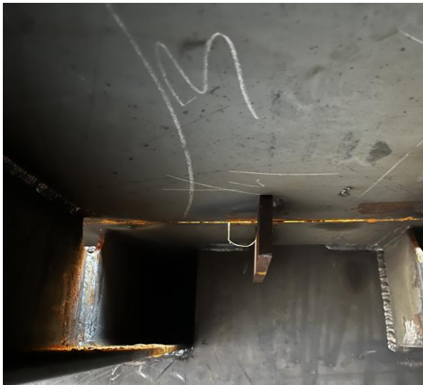
3223 – Master Butt Joint for Modules 3 & 4. Note the strongback plate holding joint in alignment.
