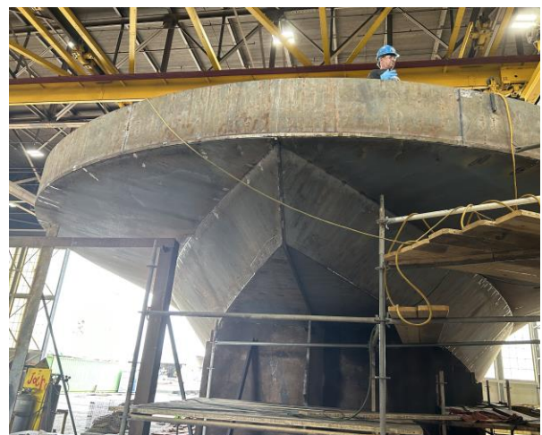
2370 – View of Module 1 from below the bow
