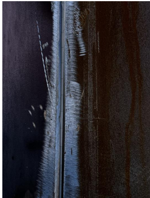
3229 – Master Butt Joint ready for welding
