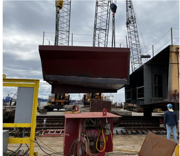
3103 - Lifting Module 2 into place on the Runway
