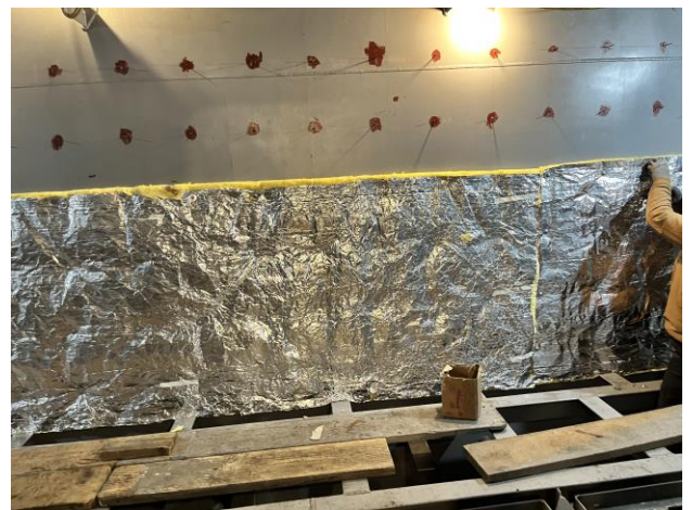
5691 - Insulating in Switchboard Room 2
