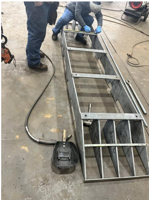
5493 – Fabricating Keel Cooler Guard
