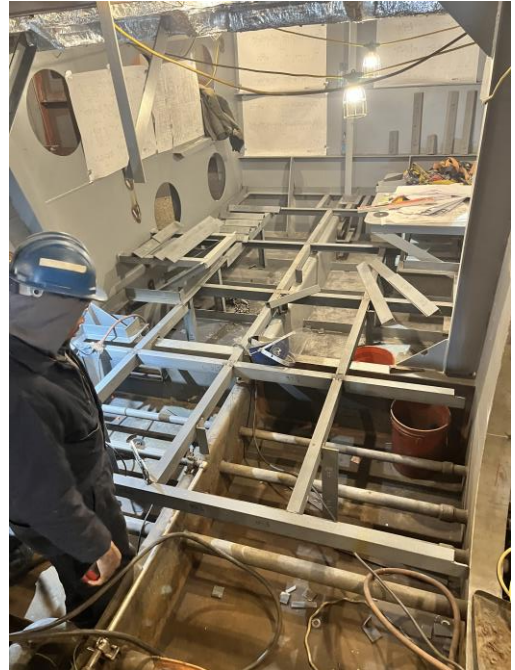
5644 – Floor Framing in Void 3
