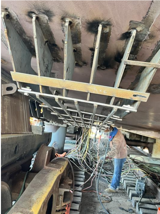
5577 – Installing Keel Cooler Guard
