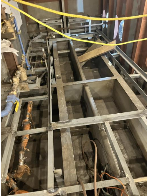
5643 – Floor Framing in Void 3
