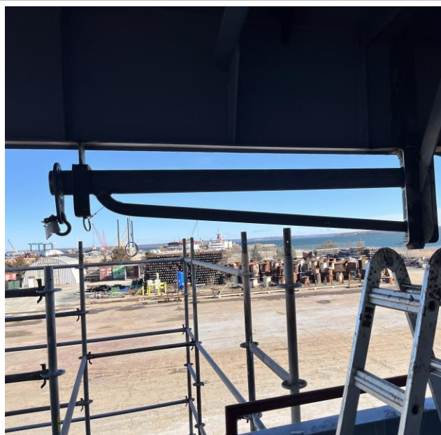
5771 – Aft Port Man Overboard Davit Installed
