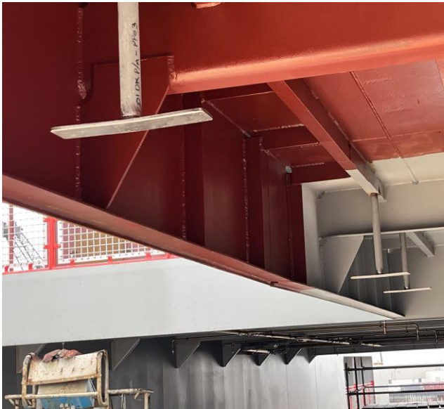
5465 – Light Supports and Partially Painted Structure
