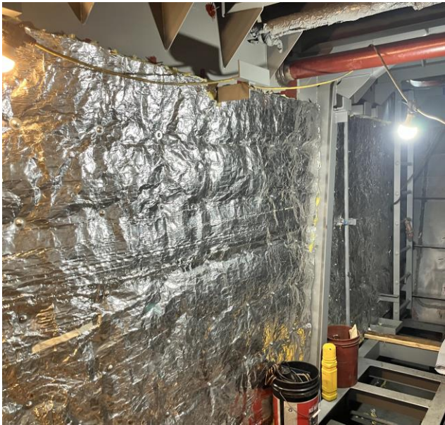
5706 – Insulating in Switchboard Room
