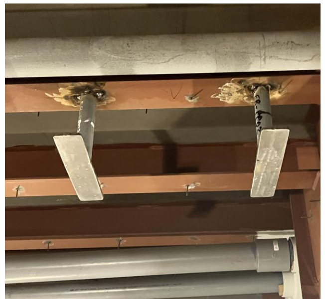
5469 – Typical Light Supports Installed
