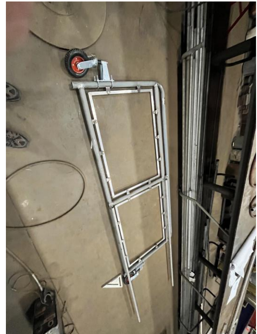
5505 – Fabricating Sliding Gate Frames
