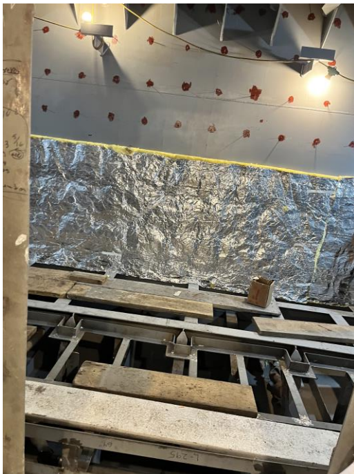
5690 – Insulating in Switchboard Room 2
