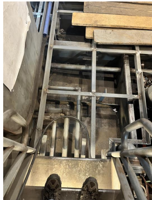
5642 - Floor Framing in Engine Rm by Stairs
