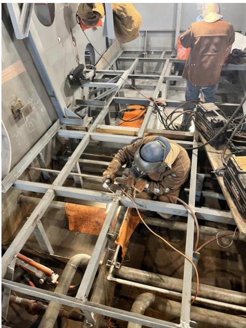
5709 – Welding on Floor Framing in Engine Room
