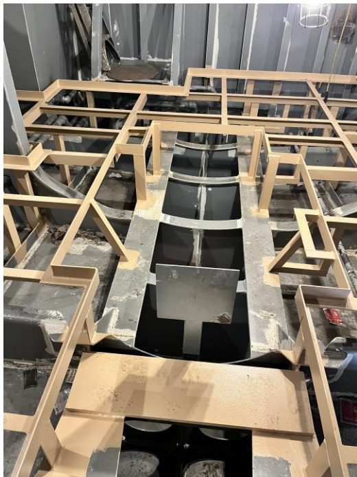
5749 – Shaft Trough in Void 2 and Floor Framing
