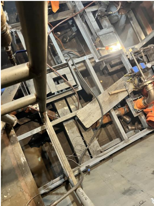
5582 – Floor Framing in Engine Rm by Stairs
