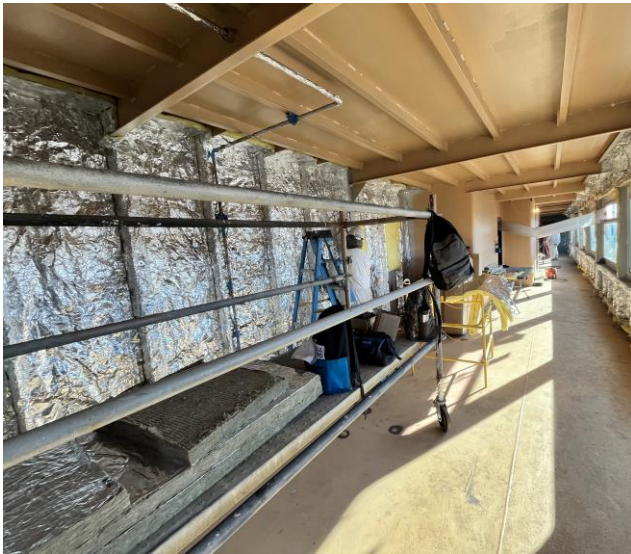
5640 – Insulating Starboard Main Deck Cabin
