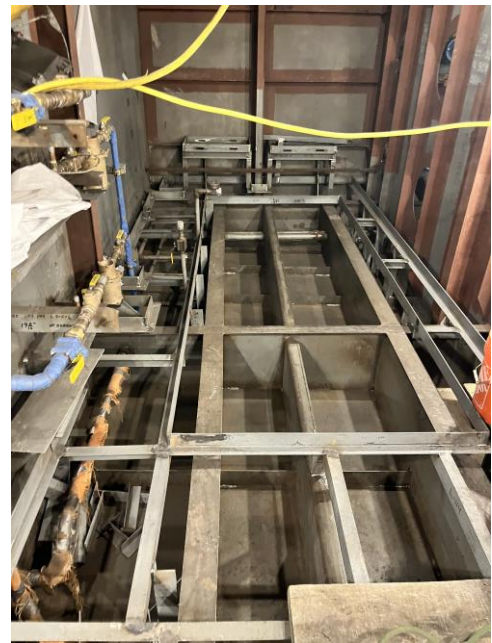
5708 – Floor and Foundation Framing in Engine Room
