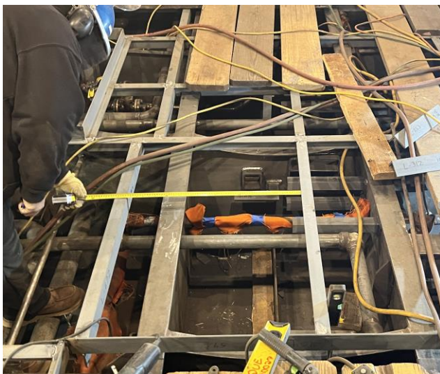
5584 - Floor Framing in Engine Rm
