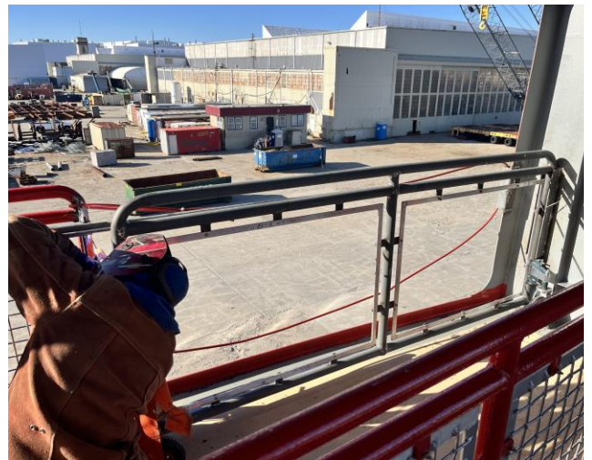
5650 – Sliding Gate installed (Starboard Aft)
