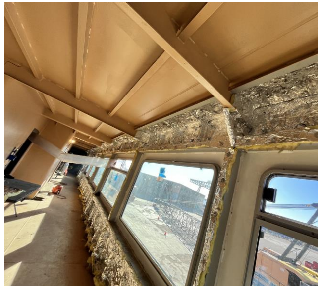
5641 – Insulating Starboard Main Deck Cabin
