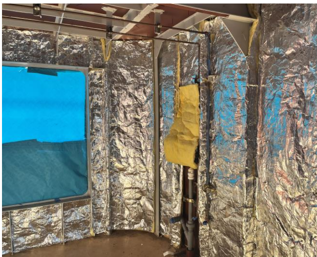
5744 – Insulation in Crew Lounge on 02 Deck
