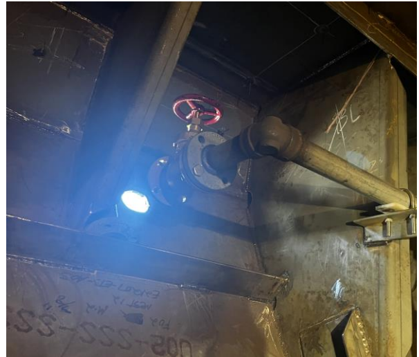
4228 – Overboard Bilge Piping in Void Space with Temporary Valve (check valve to be installed)
