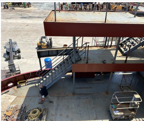
2531 – Port Stern Stairs as Seen from 02 Deck
