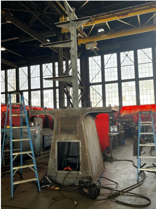
4240 – Vessel Mast Structure Under Construction
