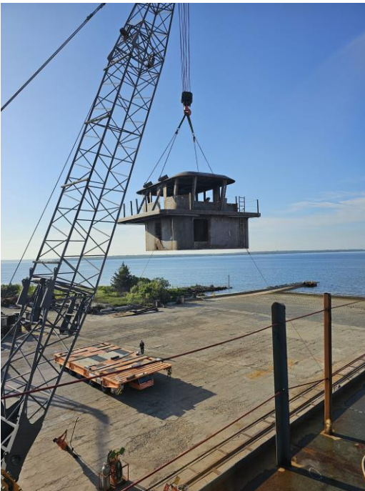
71128 – Setting Pilot House on Vessel
