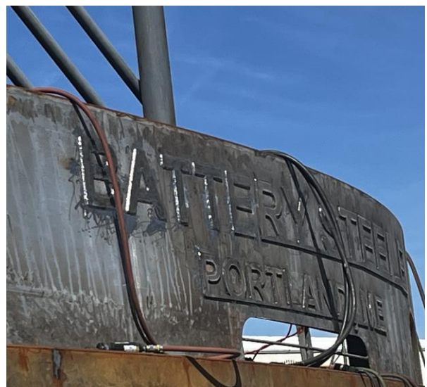
4227– Name and Hailing Port Installed
