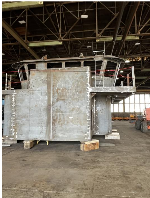
4354 – Pilot House w/Elevator Enclosure
