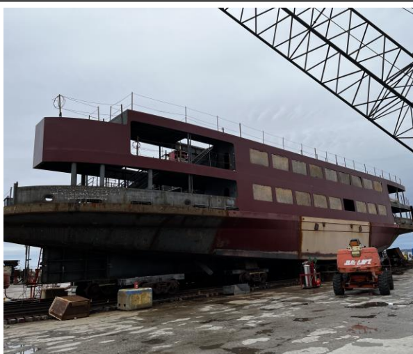
4293 – First Coat of Paint on Starboard Side
