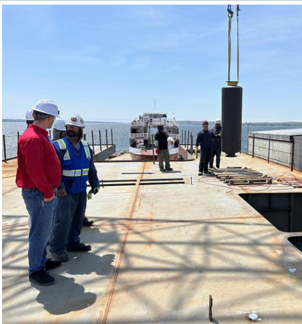
2526 – Exhaust Muffler being Placed in Vessel
