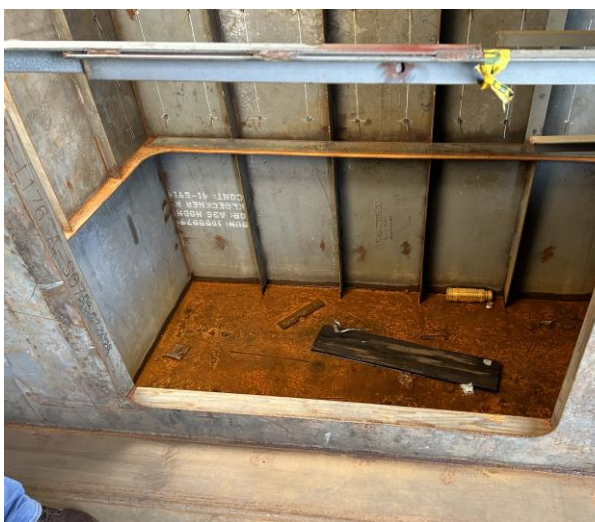
2519 – Elevator Pit at Main Deck
