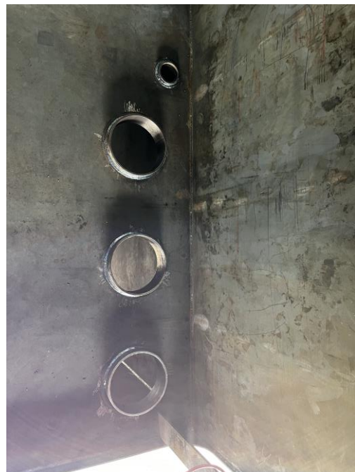
4378 – Exhaust Piping Penetrations at Pilot House
