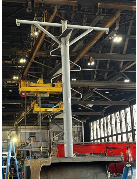
4241 – Mast on Top of Mast Structure
