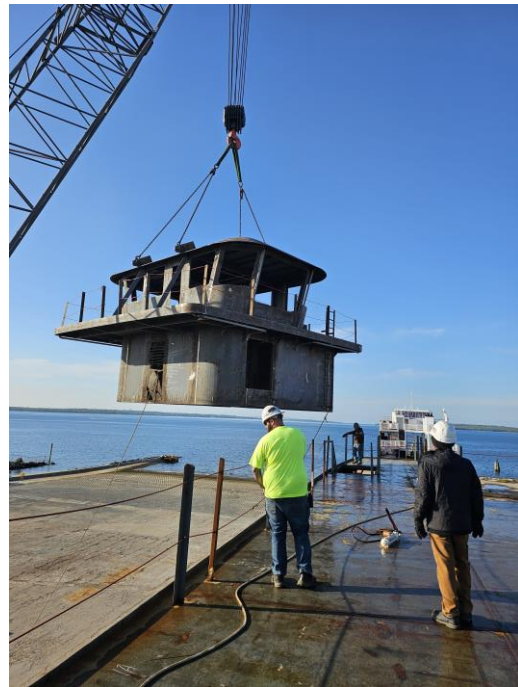
71226 - Setting Pilot House on Vessel
