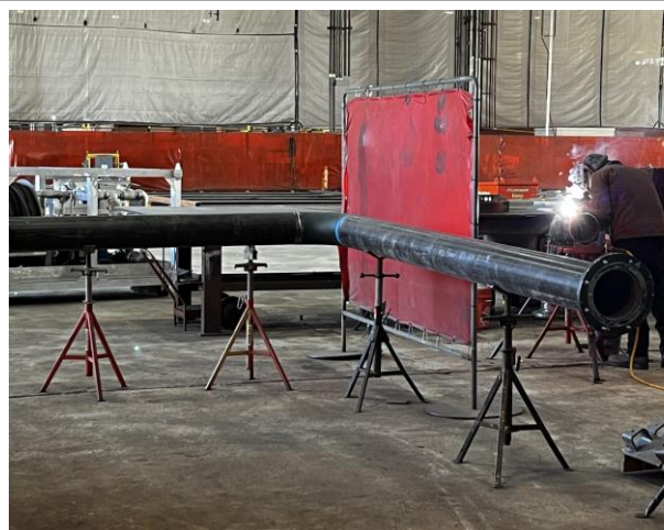
4386 – Fabricating Exhaust Piping Sections
