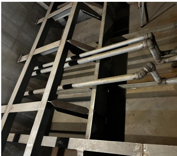
4391 – Bilge Piping under Equipment Foundation Framing
