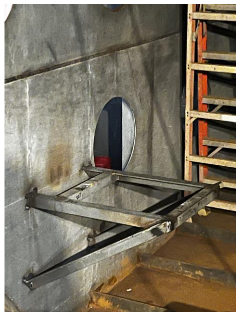
4349 – Auxiliary Transformer Foundation Frame
