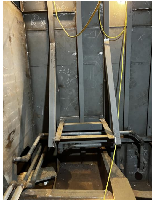
4371 – Bilge Piping and Foundation Framing
