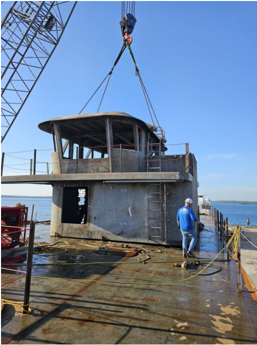
71903 – Pilot House Set in Position on 02 Deck
