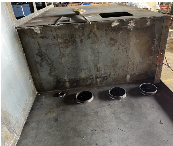
4379 – Exhaust Piping Penetrations at Pilot House
