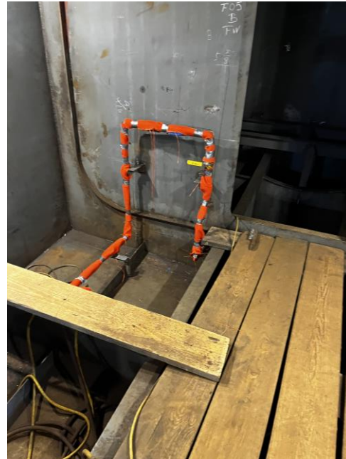
4398 – Potable Water Piping in Engine Room (wrapped for protection during construction)
