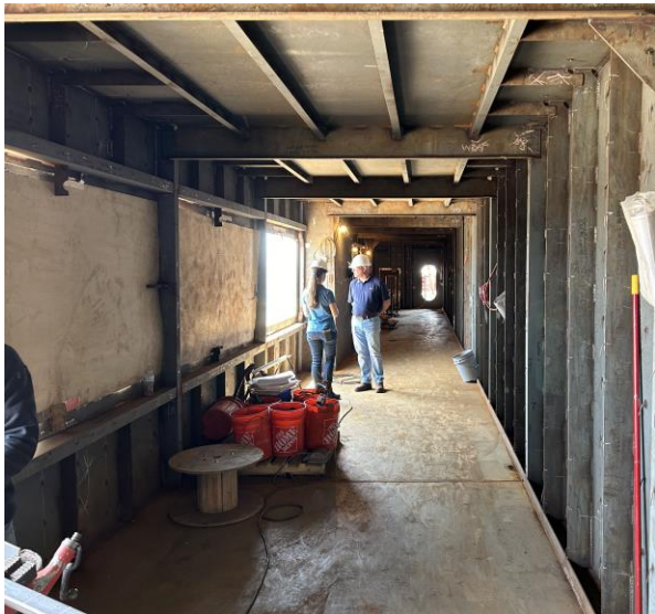
2528 – Looking Down Port Cabin on 01 Deck
