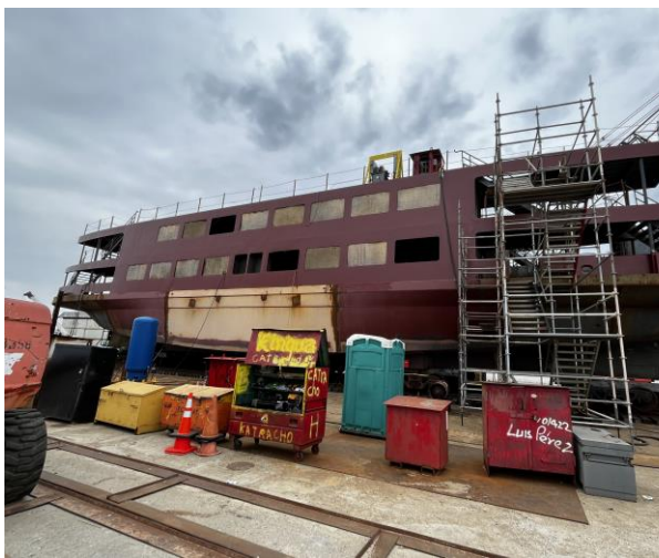
4321 – First Coat Paint on Port Side
