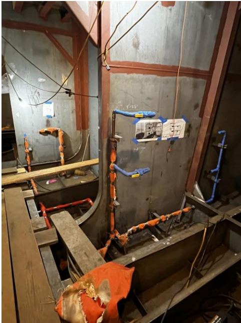
4397 – Potable Water Piping in Engine Room (wrapped for protection during construction)
