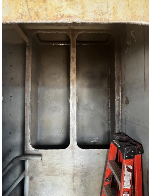
4547 – Systems Chase at Engine Room Stairs
