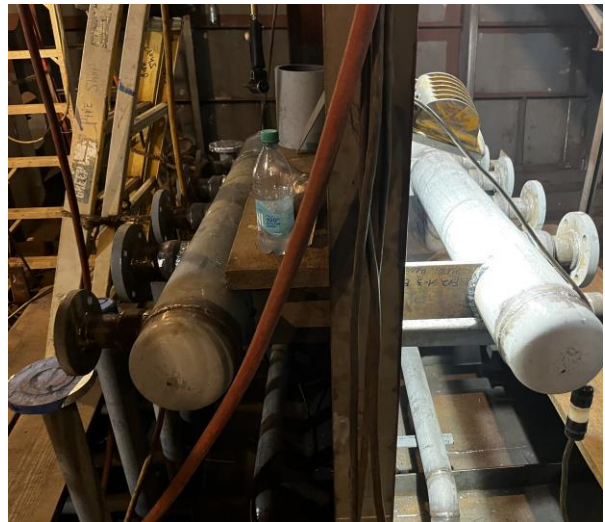
4720 – Piping Manifold Being Installed
