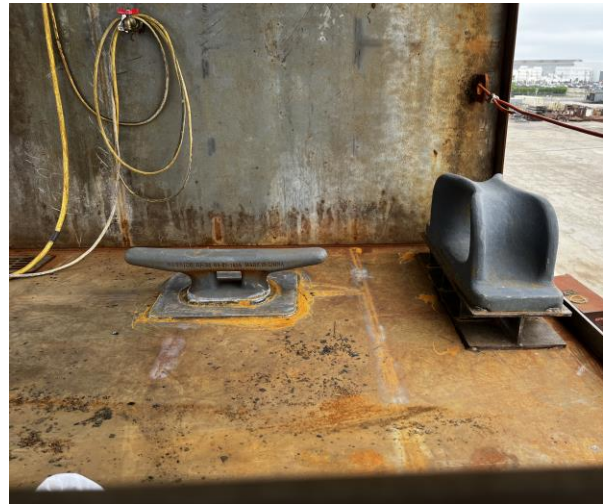
4659 – Cleat Installed & Line Chock Set & Tacked
