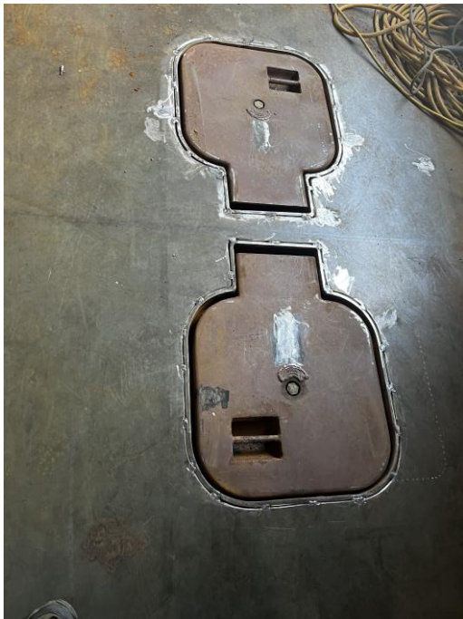
4697 – Hatches Being Installed
