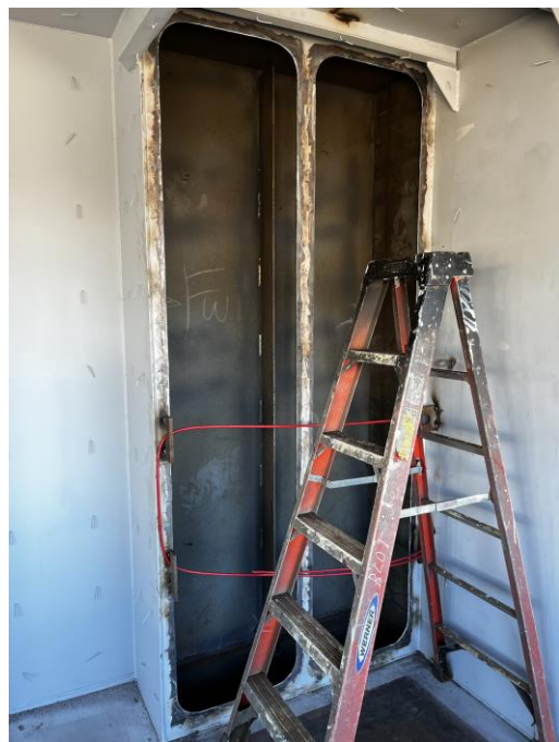
4570 – Systems Chase on 01 Deck
