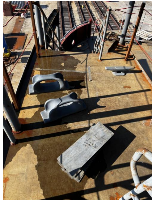
4568 – Line Chocks and Cleat Ready for Installation
