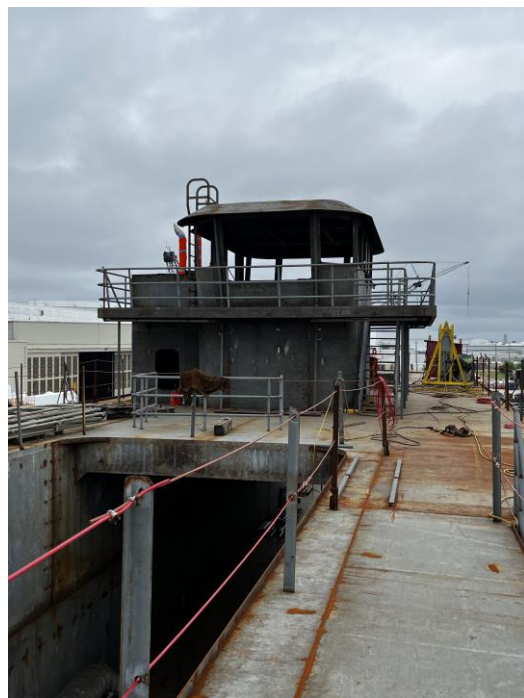
4657 – Handrail Installed Around Pilot House
