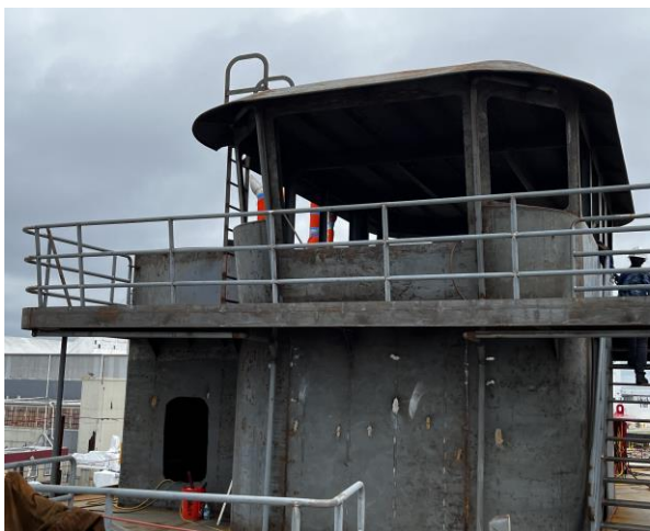
4655 – Handrail Installed Around Pilot House
