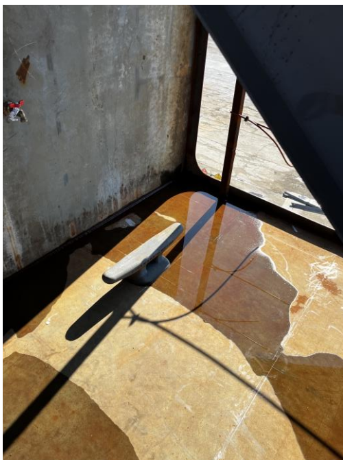
4569 – Cleat Install Location
