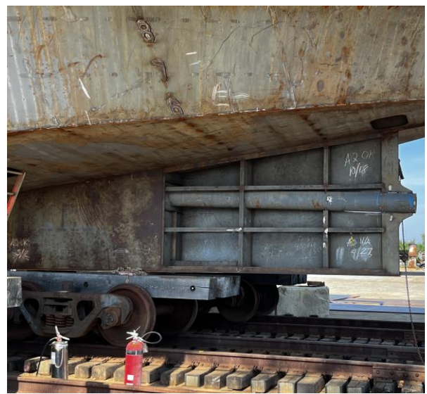
4621 – Stern Tube Being Installed, Bow End
