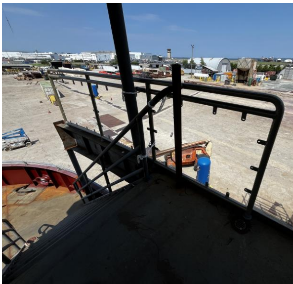
4721 - Pedestrian Handrail System being Installed
