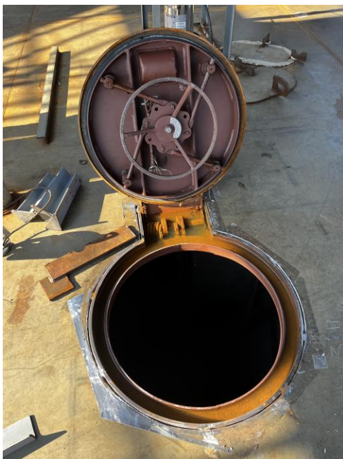
4715 – Hatches Being Installed
