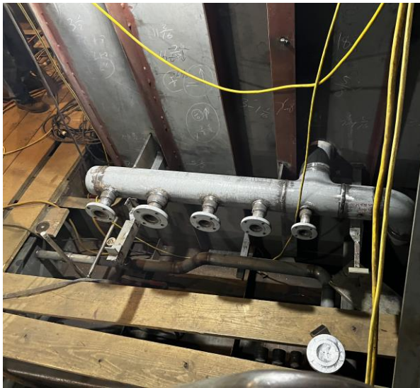
4718 – Piping Manifold Being Installed
