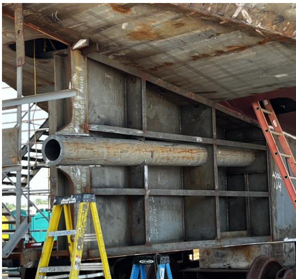
4618 – Stern Tube Being Installed, Stern End
