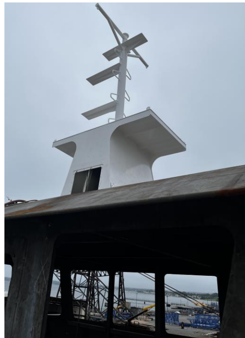
4765– Mast on Pilot House
