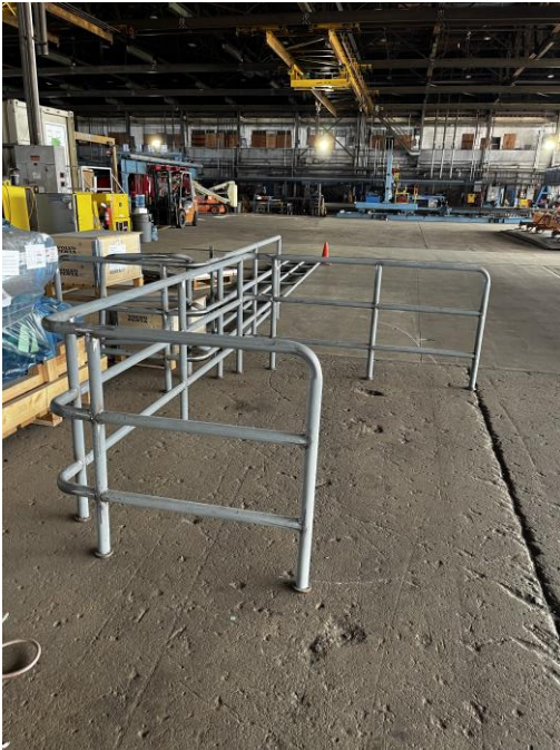
4619 – Handrail Sections Assembled and Primed
