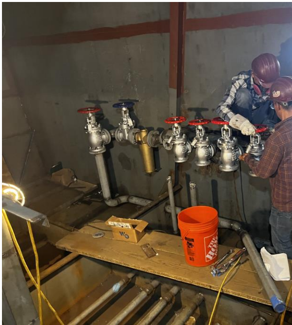
4750 – Valves Being Installed on Manifold
