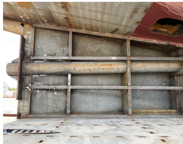
4676 – Stern Tube Installed
