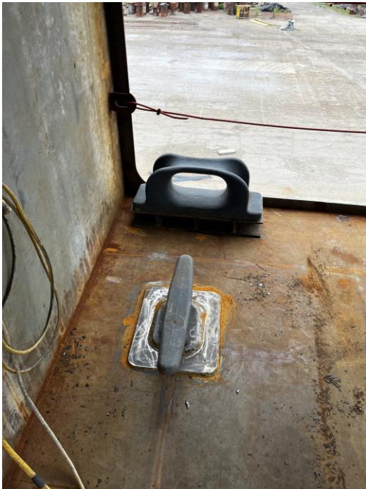
4658 – Cleat Installed & Line Chock Set & Tacked
