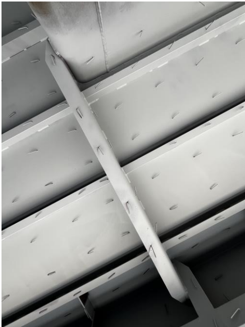
4508 – Paint & Insulation Pins, Main Deck Starboard Cabin
