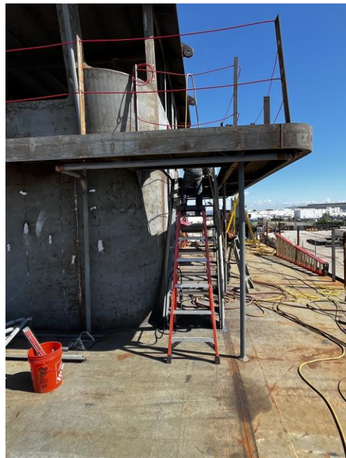
4536 – Stair Access to Pilot House
