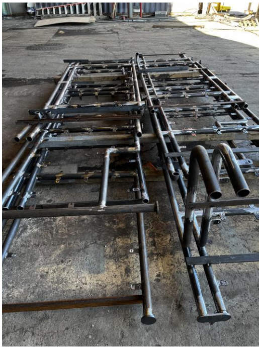
4577 – Handrail Sections Fabricated
