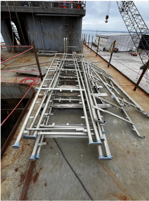
4652 – Handrail Sections Assembled & Primed
