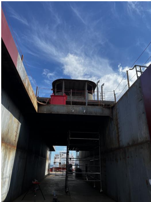
4556 – View Down Center of Vessel from Stern
