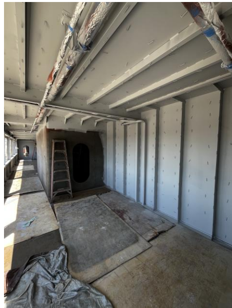
4509 – Paint & Insulation Pins in Main Starboard Cabin @ Elevator Opening, Insulated Piping Overhead
