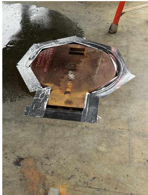
4704 – Hatches Being Installed
