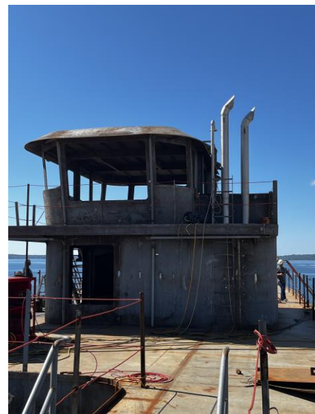
4542 – View of Pilot House from Stern, note exhaust stacks in for generators and sewer tank vent pipe
