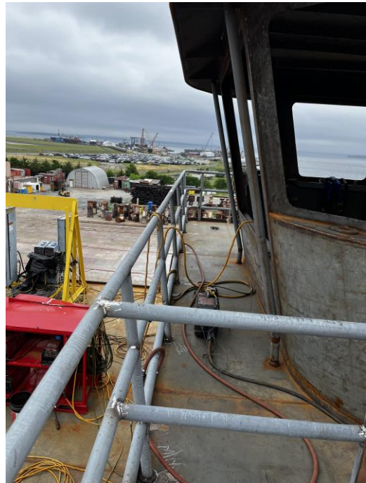
4653 – Handrail Installed Around Pilot House
