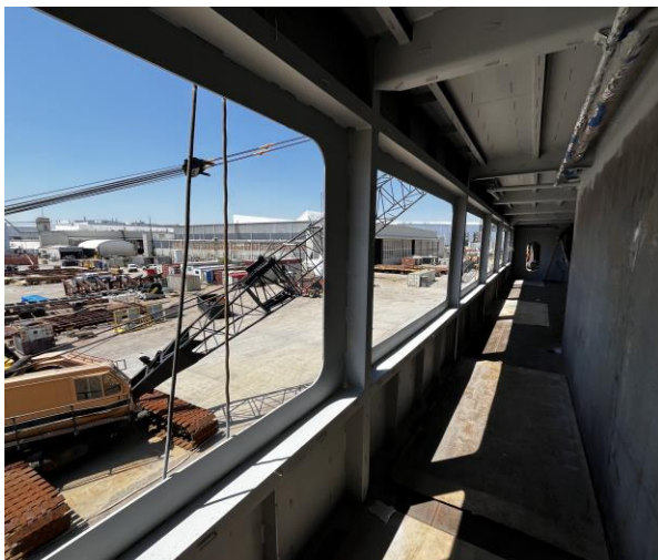
4510 – Paint & Insulation Pins in Main Starboard Cabin @ Elevator Opening, Insulated Piping Overhead
